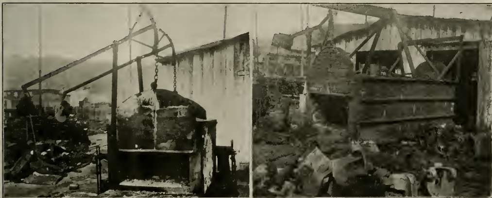
HEATING FURNACES, VIRGINIAN RAILROAD RECLAMATION PLANT.
